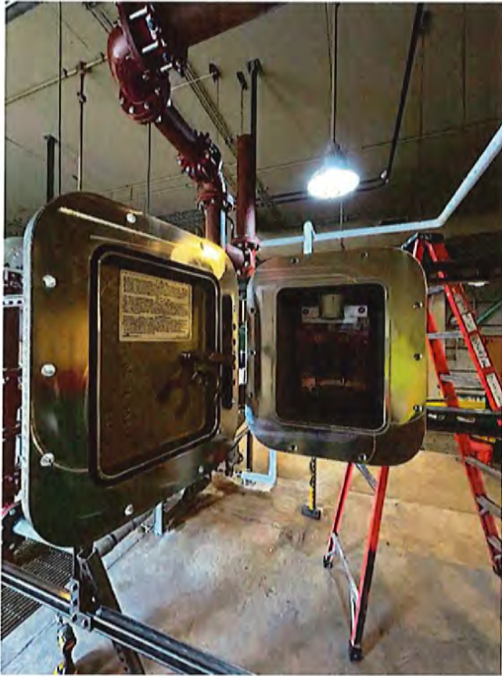
Figure 3 - New electrical panel at Grit System
