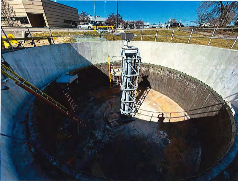
Figure 1-Clarifier No. 2. Concrete repairs nearly complete and mechanical equipment being installed.
